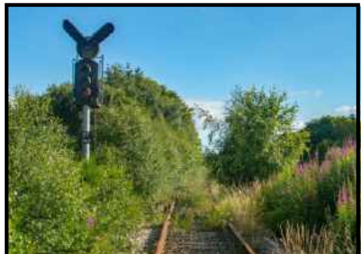
Signal ET568 still controls exit from Levenmouth at Thornton North Junction
